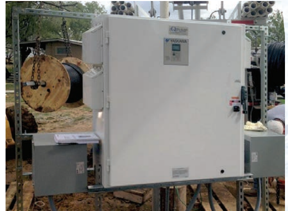
20 HP Submersible Pump Control for Irrigation.
